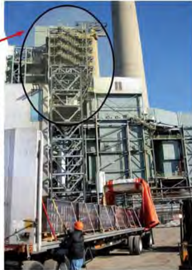
Selective catalytic reduction (SCR) systems are a means of reducing the nitrogen oxide emissions of power generators. Figure shows the typical design features and location of an SCR catalyst reactor installed in a coal-fired power plant.
